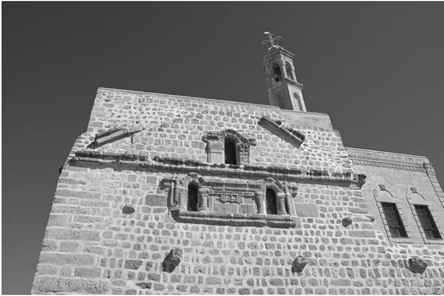
Fig. 3.2.18 West façade of the Church of Mor 'Azo'el at Kfarze
